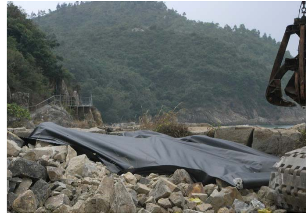
Photo 2 - Tarpaulin sheets were observed to have been used to cover excavated materials for the part that was not actively used.
